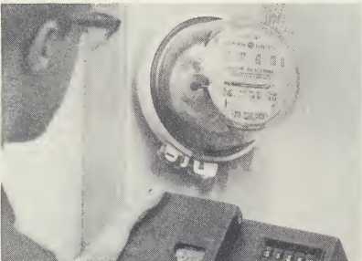
Account or meter number and meter reading being recorded.
